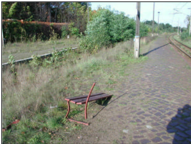
The platform still in use at the Caputh-Geltow station (federal state of Brandenburg)
