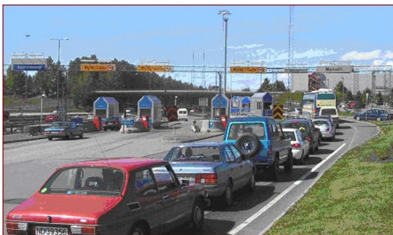
The Oslo toll-ring, showing manual toll booths and automatic gates on the E-6 motorway.
